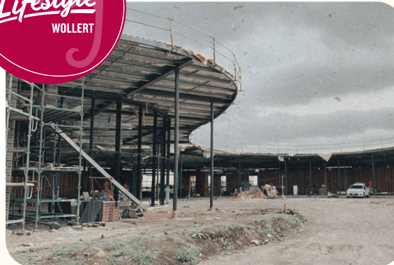
First frames underway and clubhouse under construction
