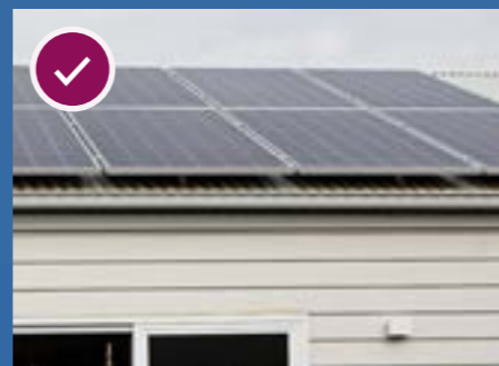
2.2kw solar panel system
